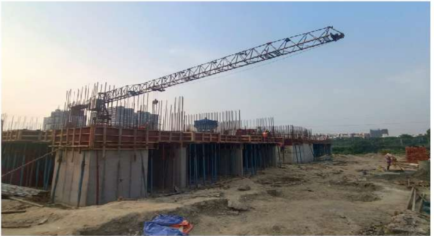
TOWER -2, SLAB SHUTTERING WORK IN PROGRESS.
