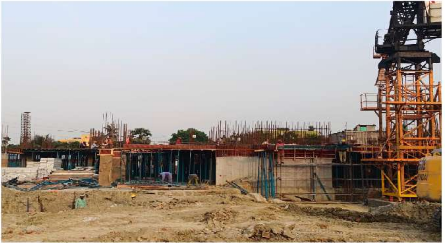
TOWER- 2, 1ST FLOOR SHUTTERING AND REINFORCEMENT WORK IN PROGRESS
