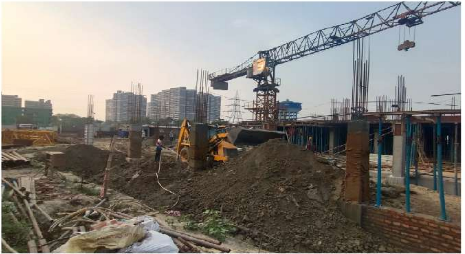
PODIUM PORTION EARTHFILLING WORK IN PROGRESS
